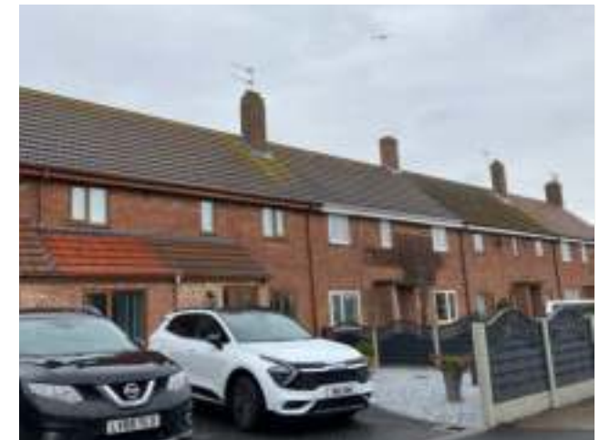
Figure 23: Terraced housing on Church Road.
